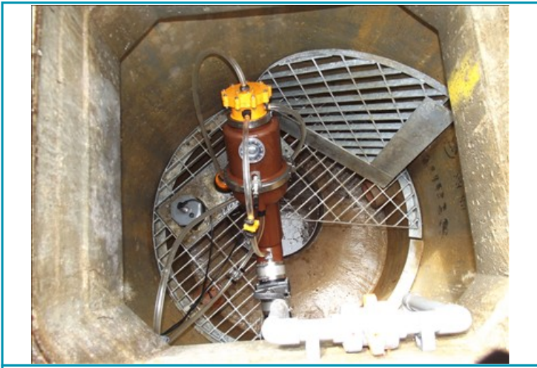
Sewage company owned pumping sump located in neighbours rear access driveway.
